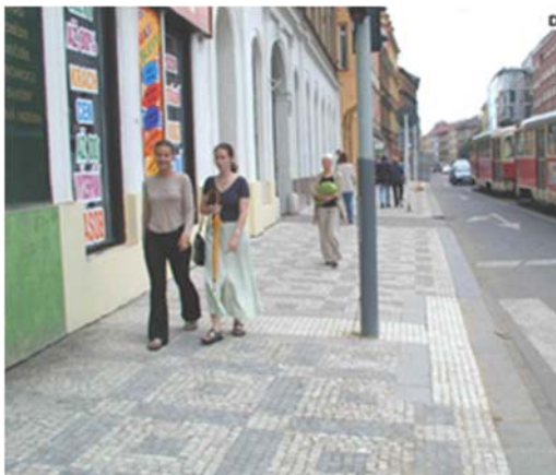
Figure 49: Natural Border Line (building), Signal and Warning Strap at a Crossing (Czechia)
