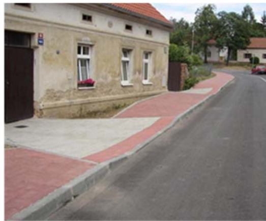
Figure 50: Dropped Kerbs on the Pavement and Contrasting Material (Czechia)
